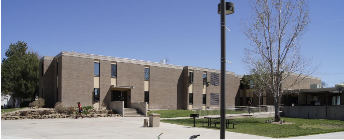
Wunsch Hall 1966 -remodeled 2001-2015: Interior remodels only have occurred. Exterior might need CHS review.
